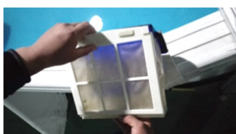
4. Move the filter panel outwards about 2 cm
